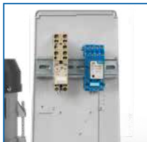
Standard DIN rail, installed behind the control board panel for mounting relays and other accessories
